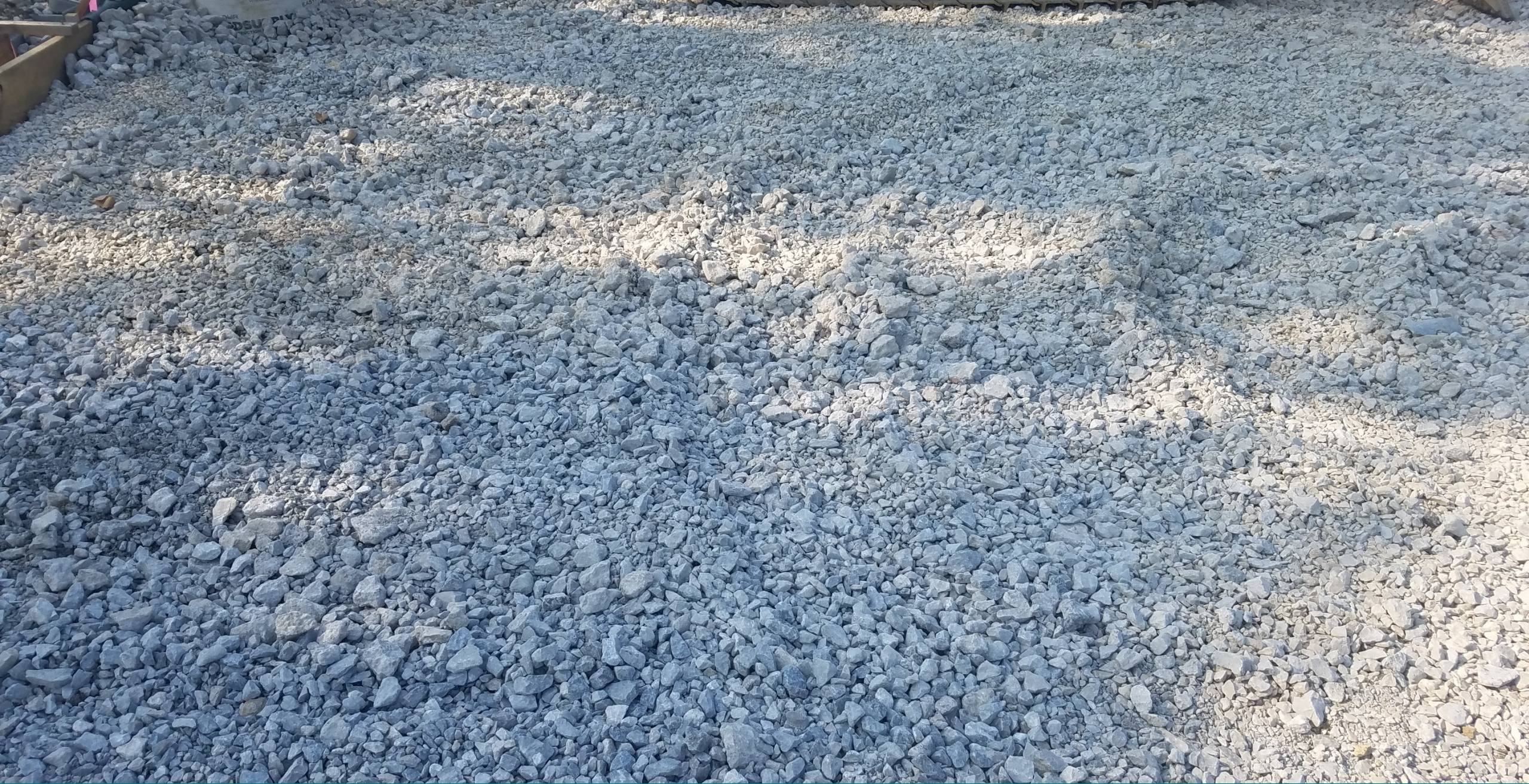
Construction: Aggregate Sub-base
