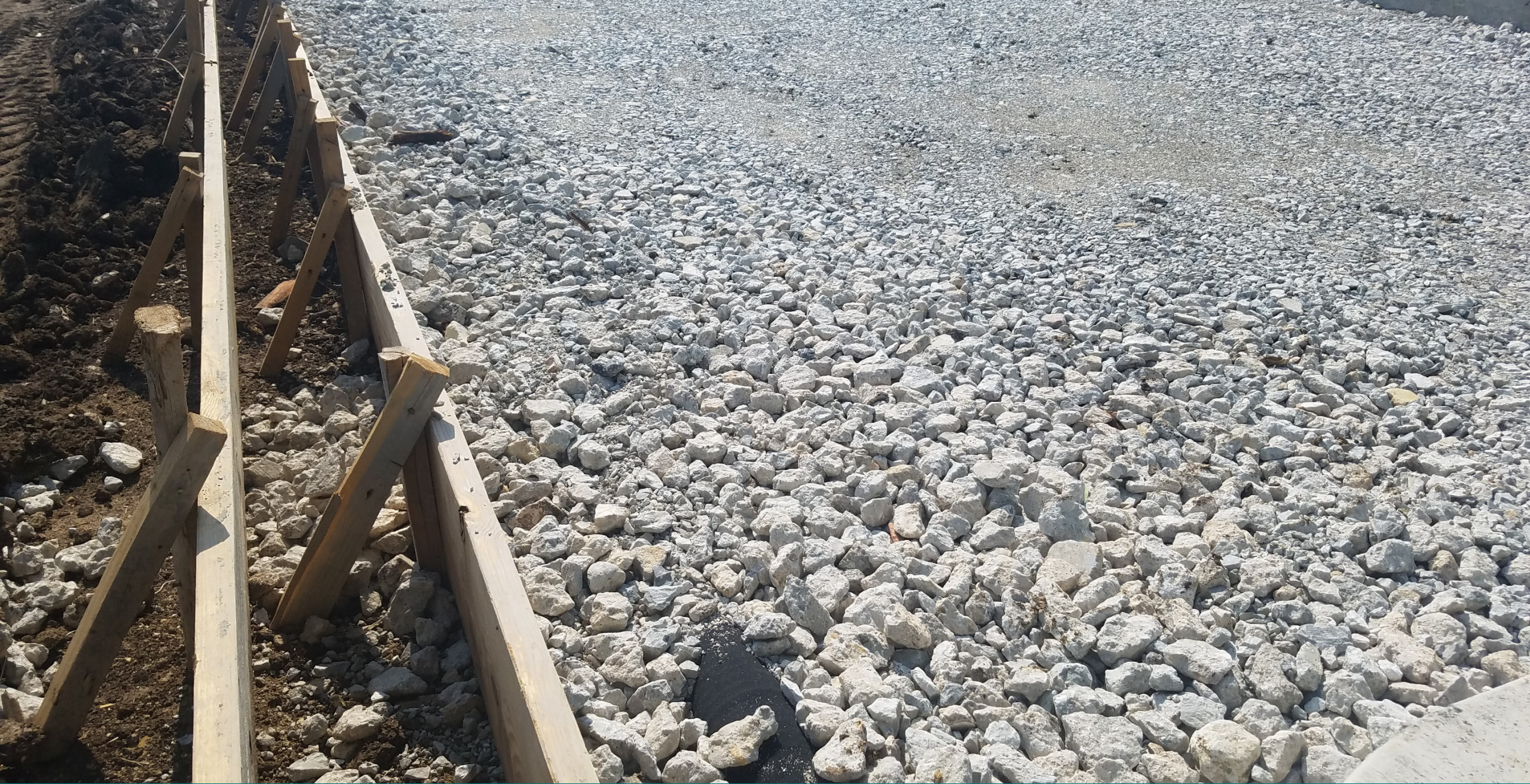
Construction: Aggregate Sub-base
