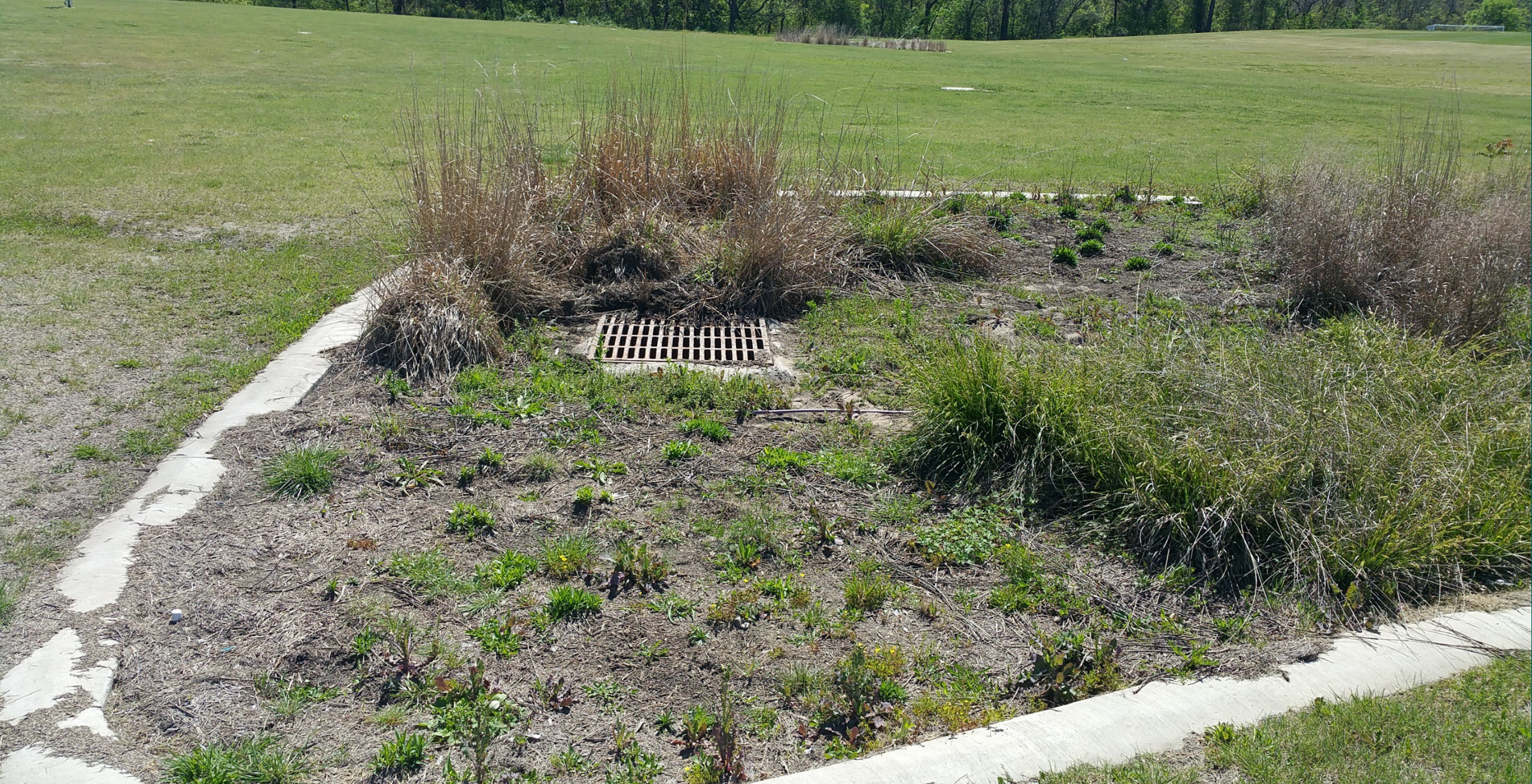
Maintenance: Clogged Bioretention Cells
