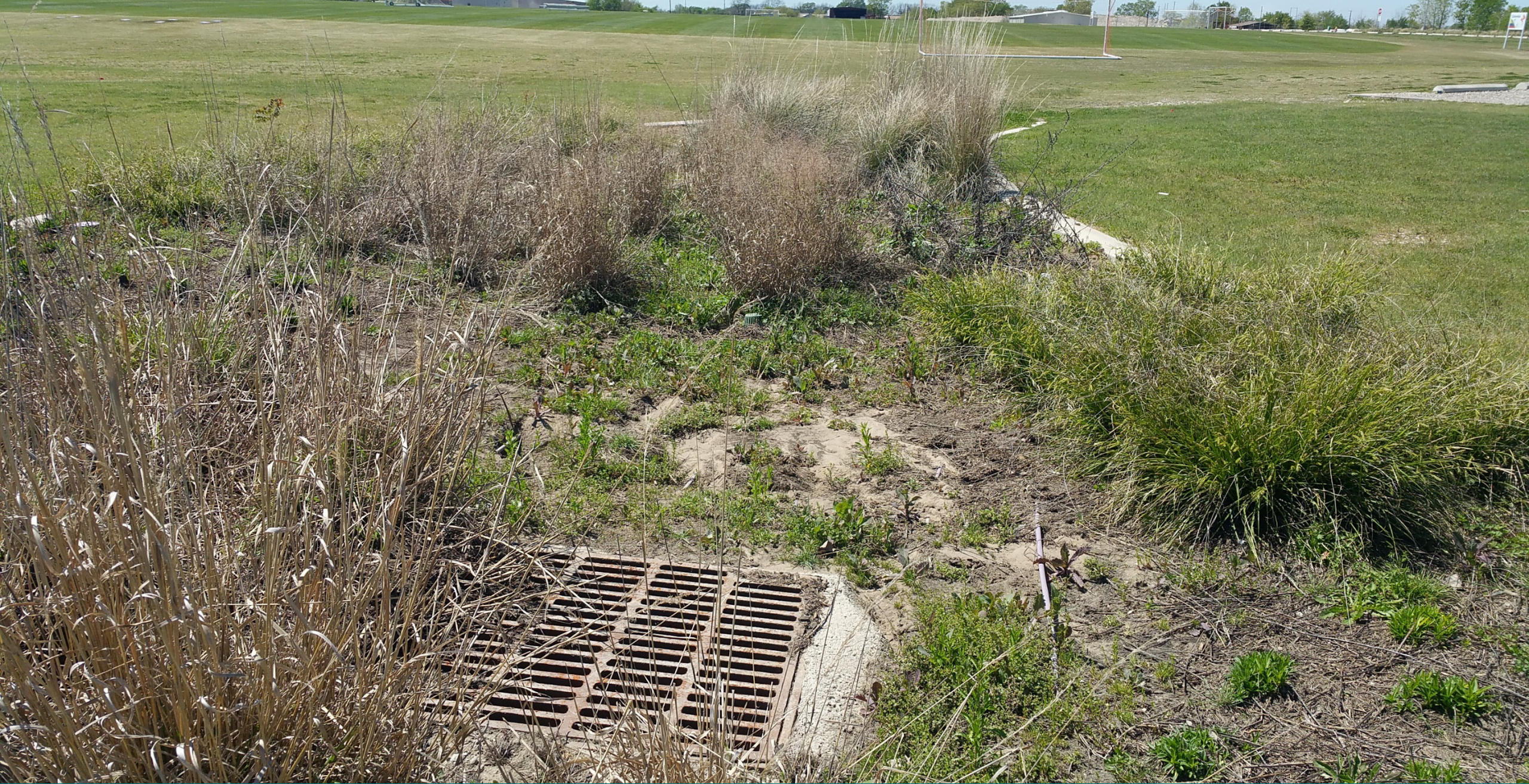
Maintenance: Clogged Bioretention Cells
