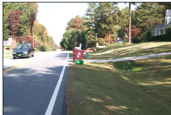
**Figure 2.31 Using Vegetated Swales Instead of Curb and Gutter**
