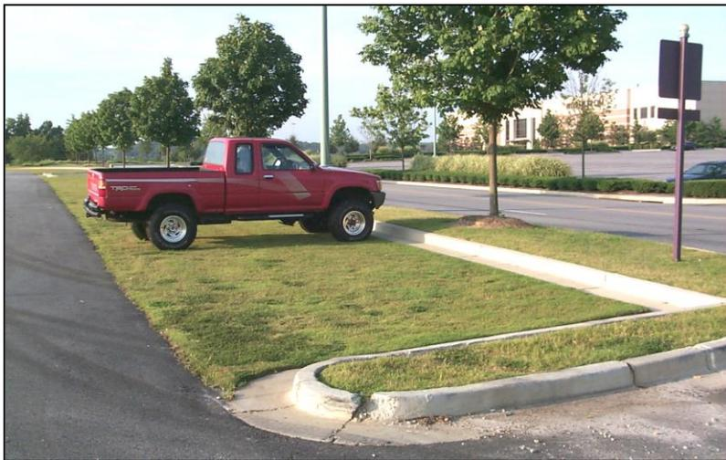
**Figure 2.22 Grass Paver Surface Used for Parking**
