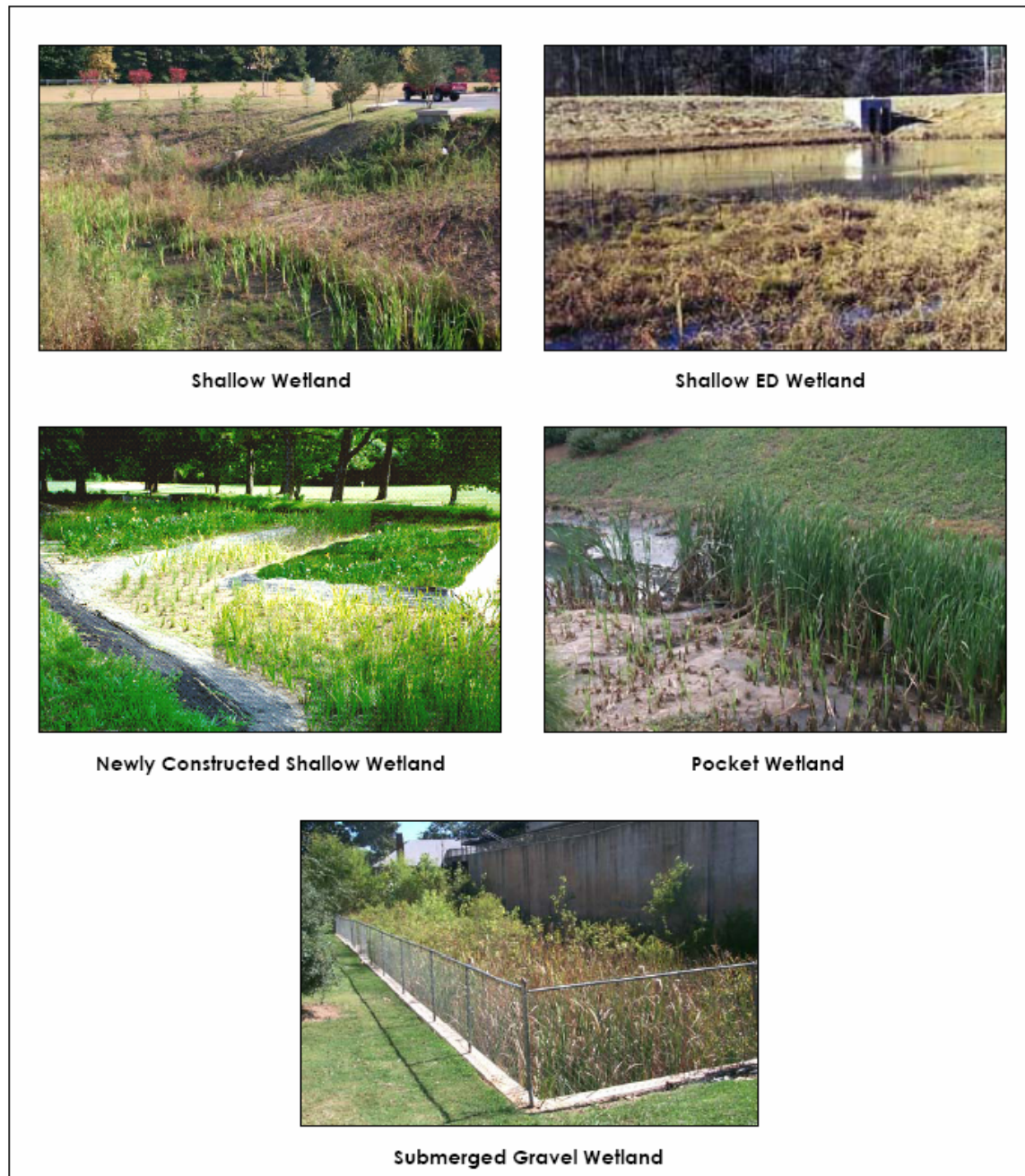
Figure 5.2.27-1 Storm Water Wetland Examples
