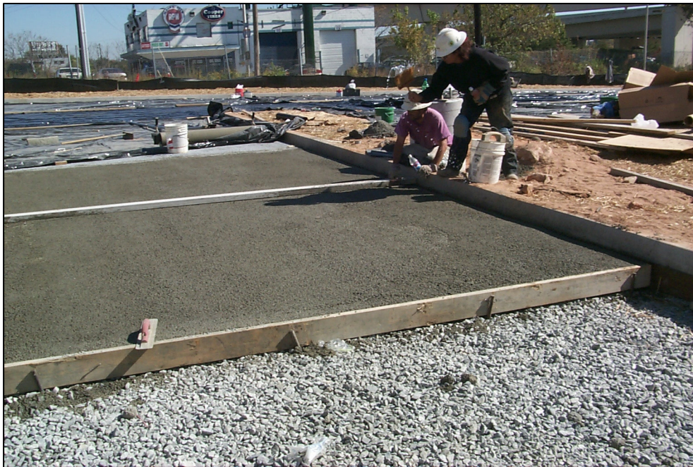
Figure 5.2.24-2 Porous Concrete System Installation
