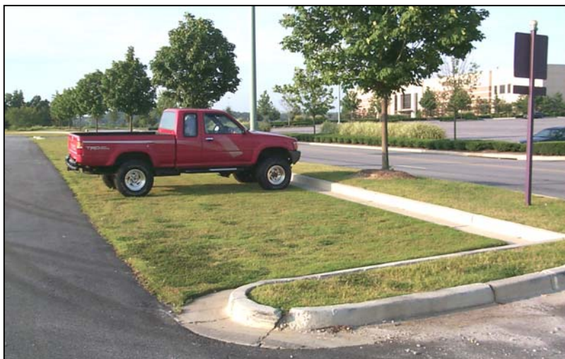
Figure 1.3.2-21 Grass Paver Surface Used for Parking
