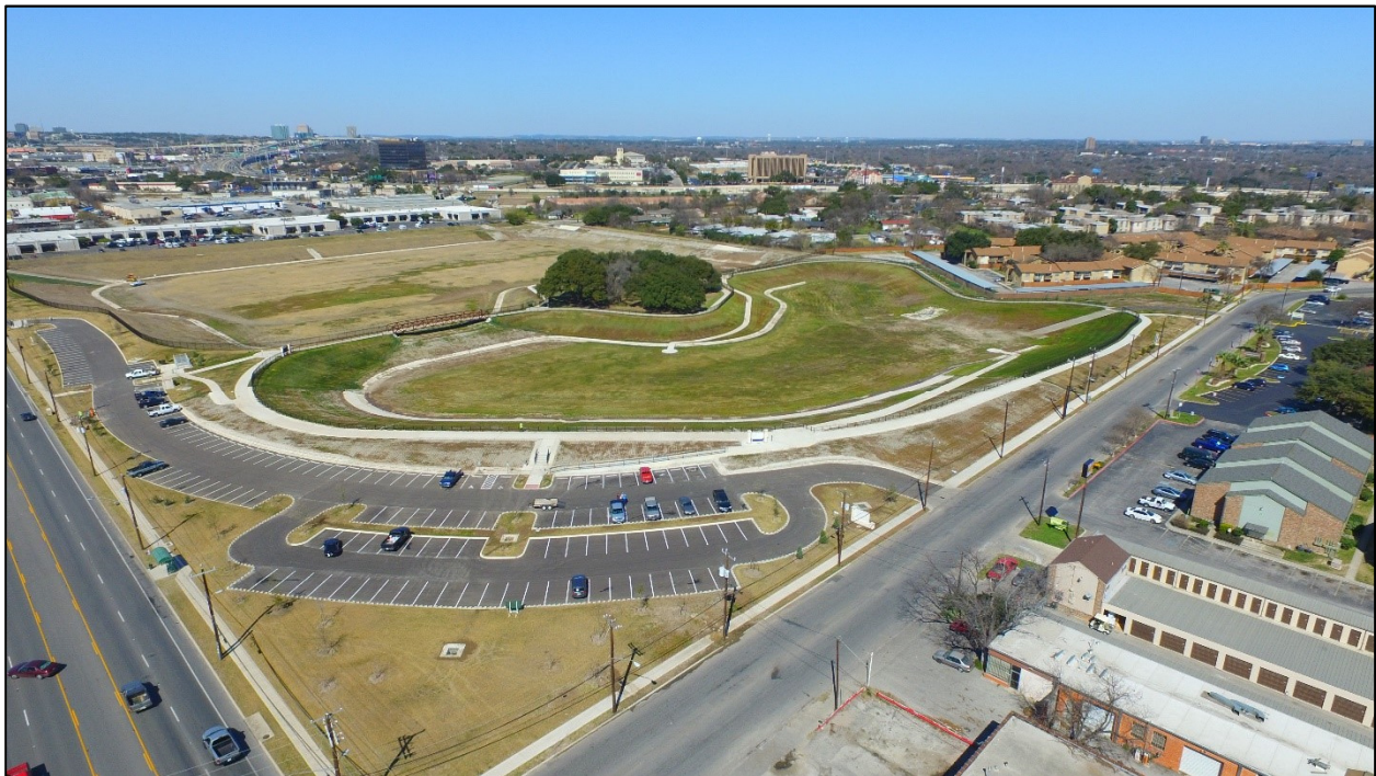
Figure 1. Laddie Place Phase III Regional Storm Water Facility resulted from a combined effort of Bexar County, the City of San Antonio and the San Antonio River Authority to convert a 28.5-acre shopping center that was almost entirely covered by impermeable surfaces except for heritage oak trees. The heritage trees are a defining feature of the former shopping mall that was converted to a regional detention facility and park with natural elements that improve the stormwater quality and increase stormwater volume.
