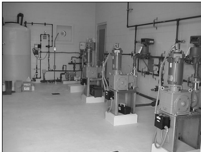
Figure 6.1 Alum Treatment System and Injection Equipment
