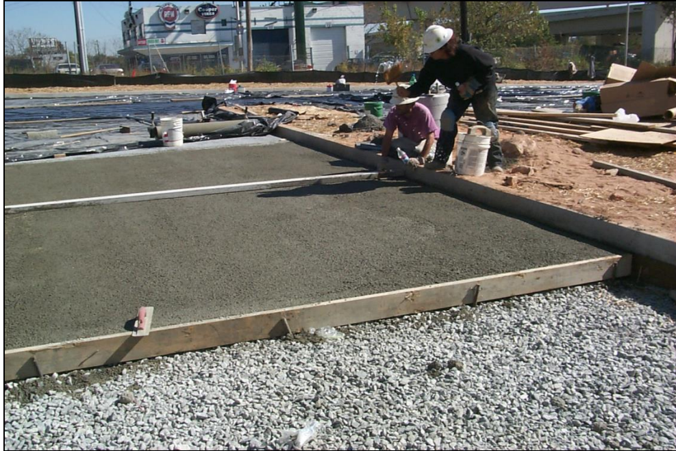
Figure 25.2 Porous Concrete System Installation
