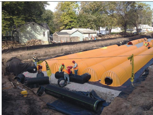
Soakage Trench installation. (Source: Wikipedia, CC BY-SA 3.0)
