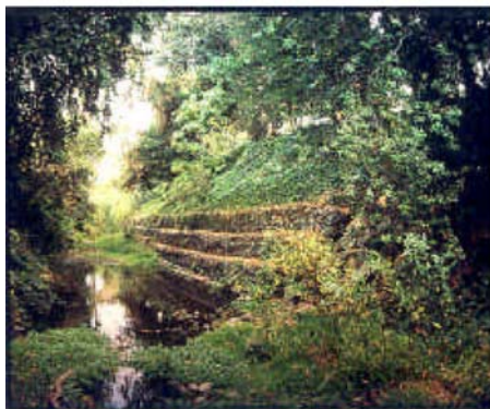
Figure 4.4-21 Gabion Baskets Installed for Slope Stabilization along a Stream
